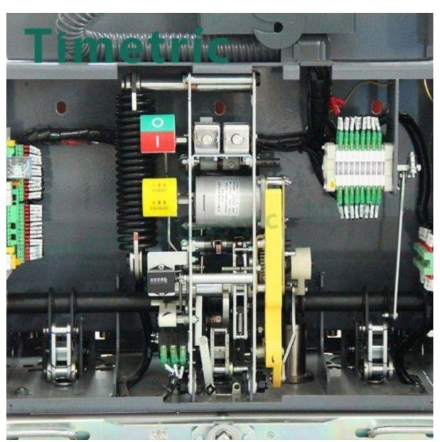
ZN63A(VS1)-12 is a HV indoor vacuum circuit breaker working as a protection and control unit of power grid equipment and industrial electric equipment in power system of rated voltage from 7.2KV to 12KV. It meets the requirements of GB/T1984-2014 (AC HV circuit breaker) and JB355-1996 (3.6KV-40.5KV indoor AC HV vacuum circuit breaker). It can be used in switchgears of KYN28(GZS1), XGN and GG-1A.
